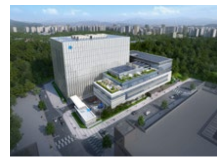
Hanam Data Center
