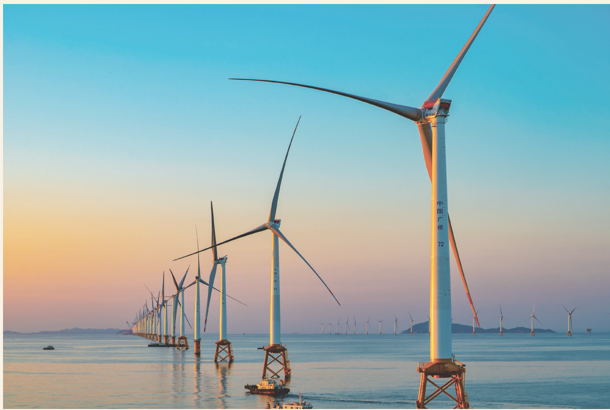
Offshore wind power project in Jiazi Town, Shanwei City, Guangdong Province
