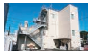
Exterior stairs to the roof
