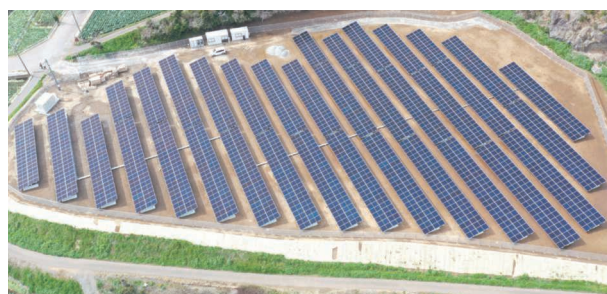
▲ Choshi Power Plant
